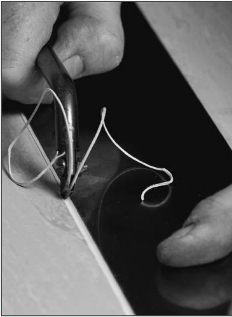
Figure 28 Grooving the seam
