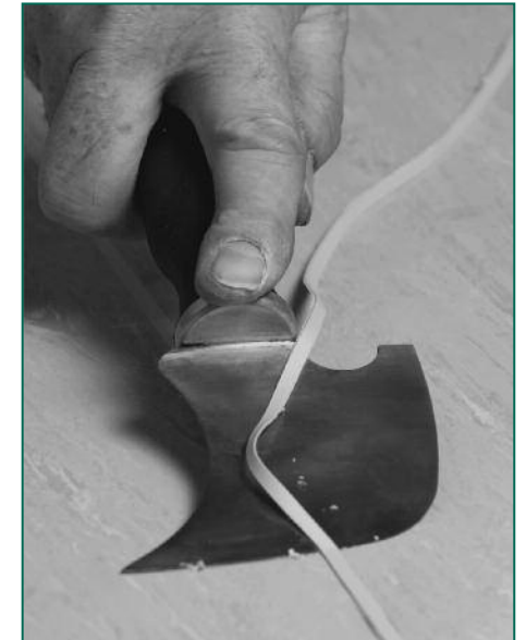
Figure 32 Final trim after the weld has cooled
