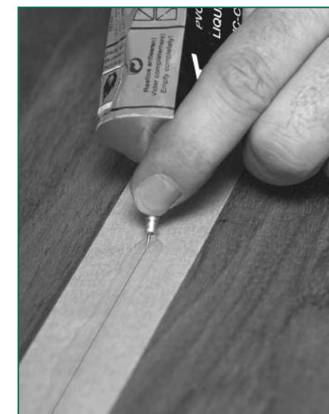
Figure 15 Cold welding
