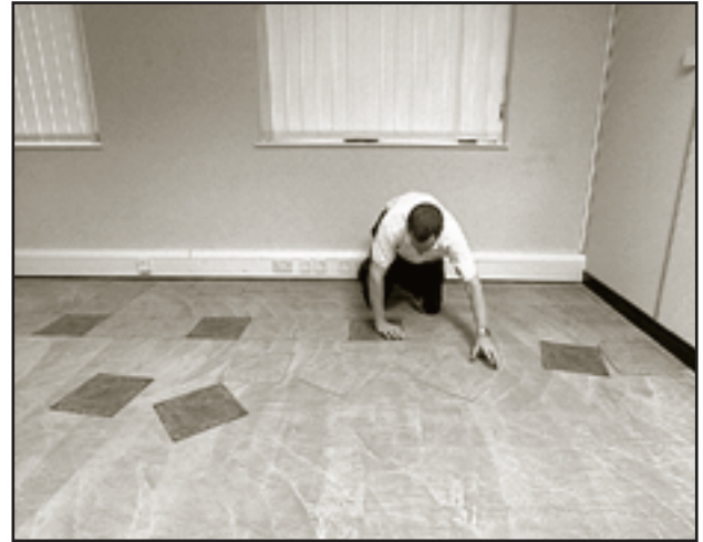
Loose lay tiles to check set out.
