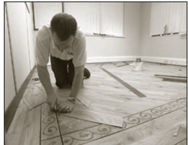
Installing border and perimeter tiles
