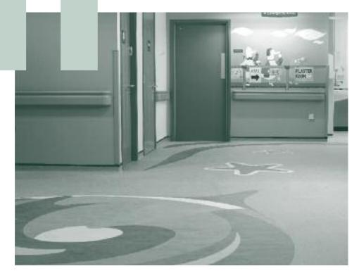
Polyflor Expressions inlaid motifs and border designs are manufactured under strictly controlled conditions to produce the close-fitting pieces which make up the design. To duplicate the close-fitting on site, it is important to ensure the design is correctly conditioned prior to laying.
