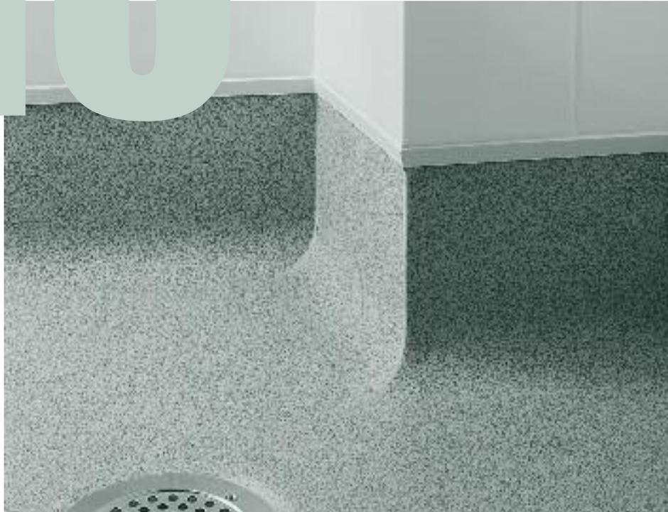
The Polyflor Ejecta ranges of flooring accessories are PVC extrusions designed for use with most vinyl floorcoverings, especially the Polyflor and Polysafe ranges. The Ejecta range includes set-in coved skirtings, sit-on coved skirtings, cove former, capping strip and CT strip as well as the weld rods covered in Welding vinyl flooring.
