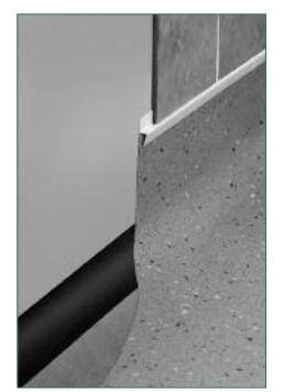
Figure 10 Fitting to ceramic tiles
