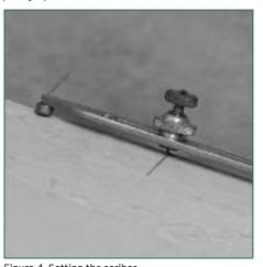
Figure 4 Setting the scriber Repeat for the other end of the sheet. Once completed, the whole sheet - when slid back into position - should fit the wall profiles exactly.
