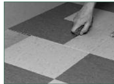
Figure 12 Measuring using an overlapping tile
