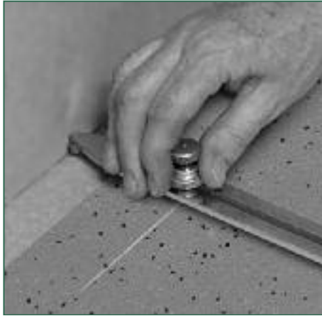
Figure 17 Scribing the wall profile
