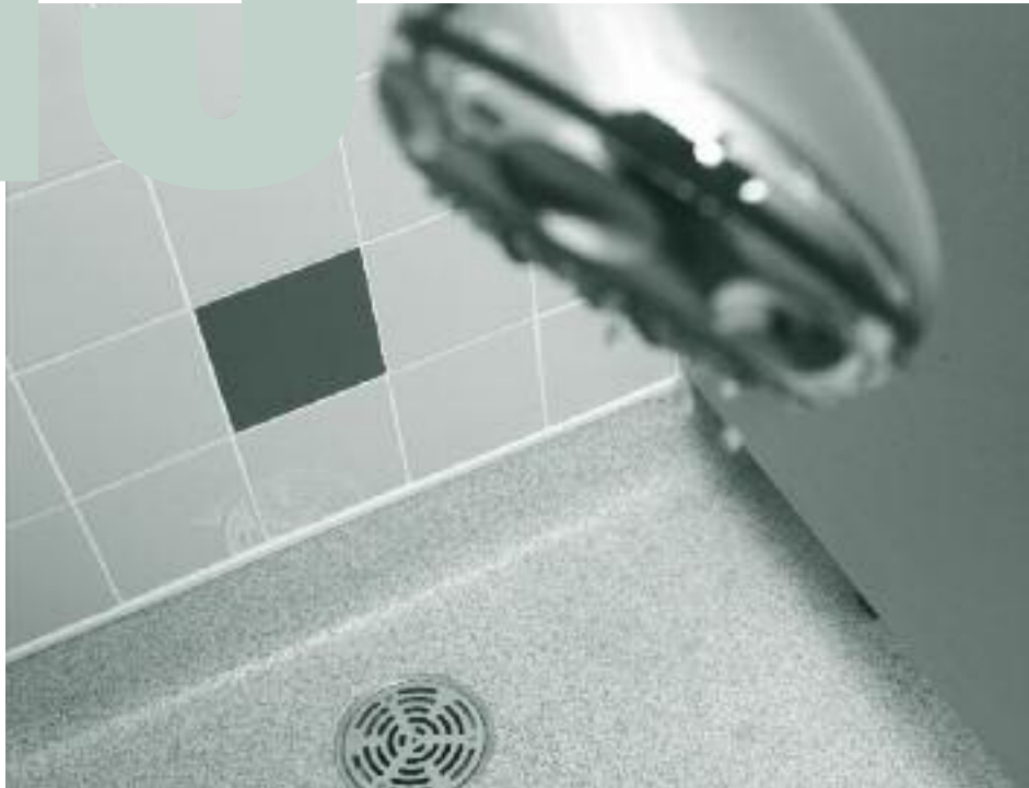
Figure 33 Stainless steel drain prior to fitting vinyl clamping ring
