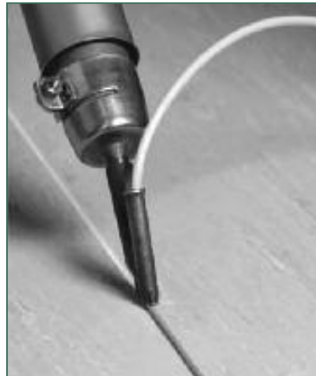
Figure 29 Applying the weld
