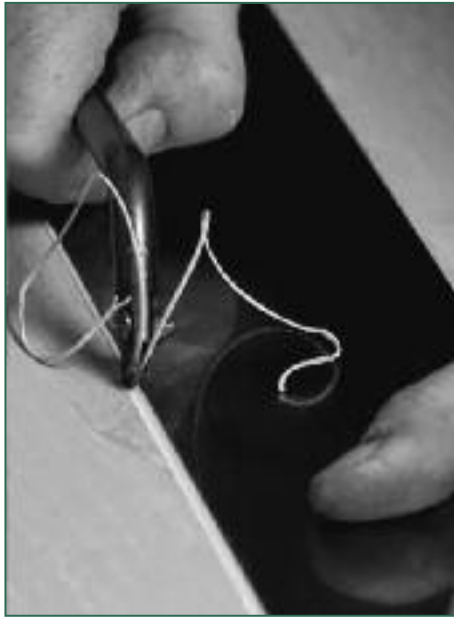
Figure 28 Grooving the seam
