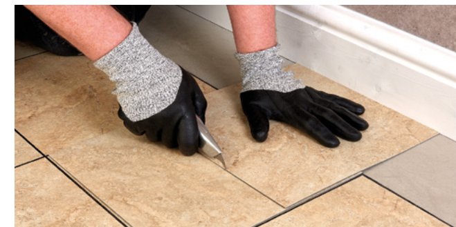
Figure 5.6 Measuring using an overlapping tile
