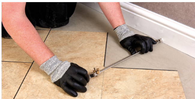
Figure 4.9 Cutting the tiles using a scribe (diagonal cut)
