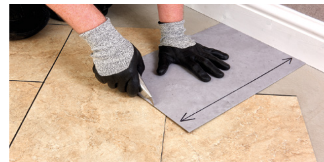
Figure 5.9 Cutting the perimeter tiles (diagonal cut)
