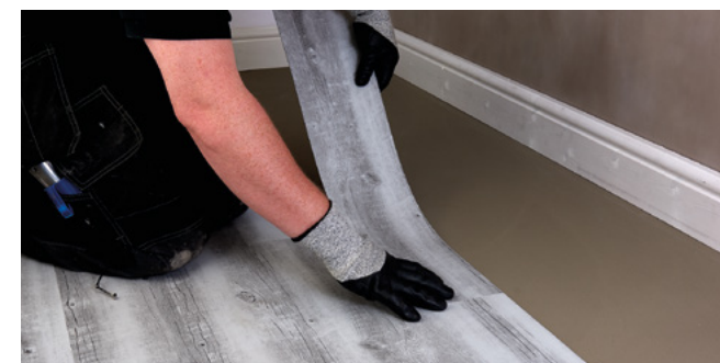
Figure 5.1 Setting planks out
