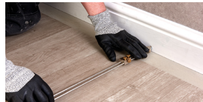
Figure 6.2 Scribing the wall profile
