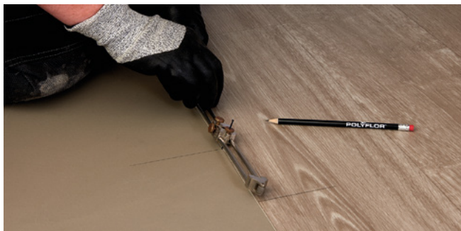
Figure 6.4 Scribing the wall profile
