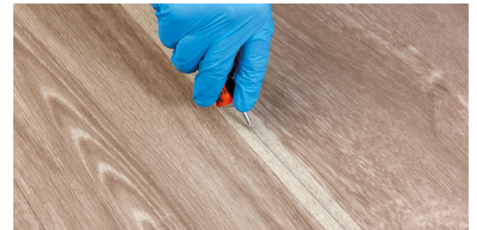
Figure 9.8 Cold welding
