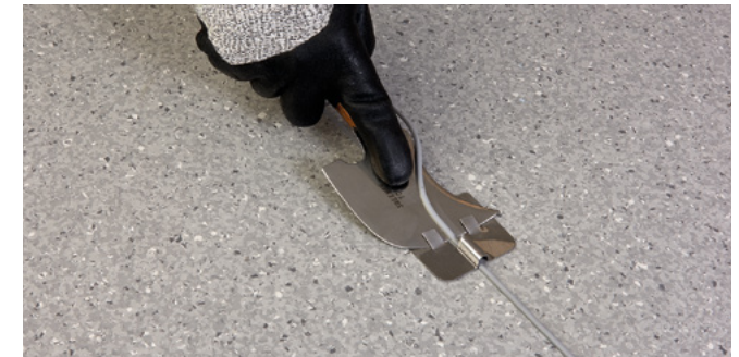
Figure 9.4a Trimming off the weld top layer (Spatula Trimming Knife)
