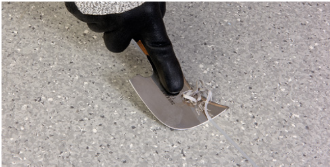
Figure 9.5a Final trim after the weld has cooled (Spatula Trimming Knife)
