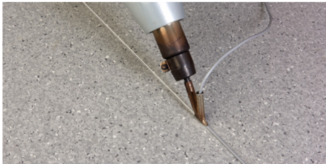
Figure 9.2 Applying the weld
