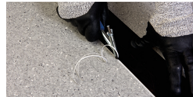
Figure 9.1 Grooving the seam
