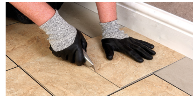
Figure 6 Measuring using an overlapping tile
