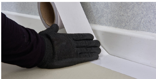
Figure 36 Use double sided QuickLay tape
