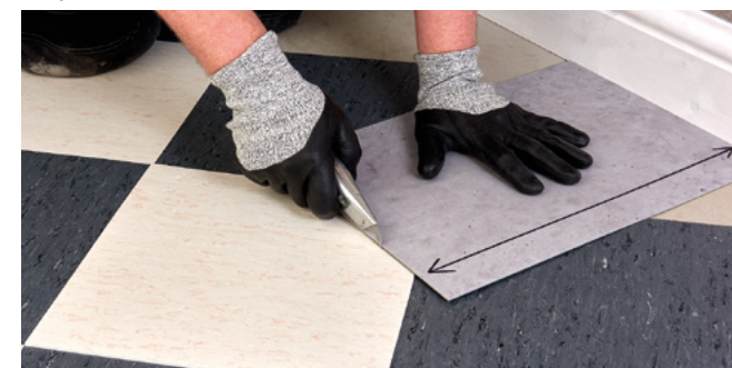
Figure 8 Cutting the perimeter tiles (diagonal cut)
