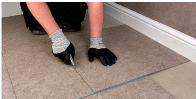
Figure 8 Measuring using an overlapping tile
