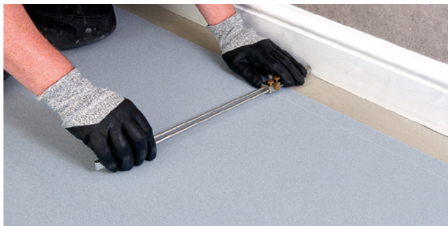
Figure 35 Scribing the wall profile
