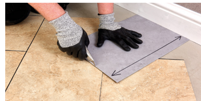
Figure 9 Cutting the perimeter tiles (diagonal cut)
