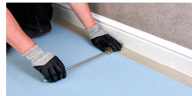
Figure 2 Scribing the wall profile
