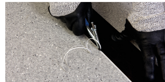
Figure 1 Grooving the seam
