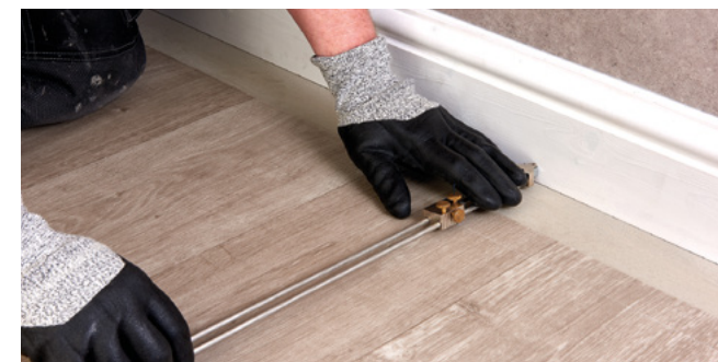
Figure 2 Scribing the wall profile
