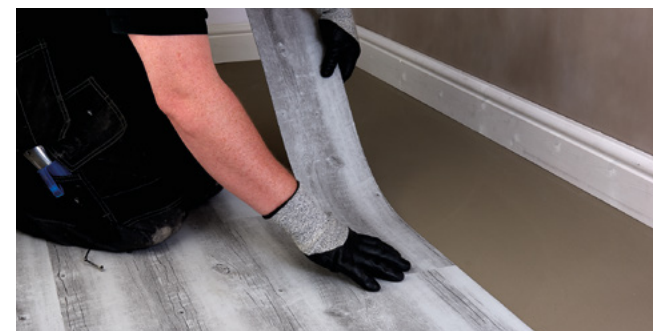
Figure 1 Setting planks out
