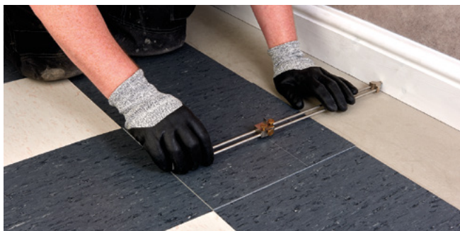
Figure 6 Measuring a tile using a scriber
