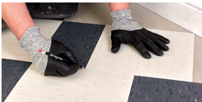
Figure 7 Marking the perimeter tiles (diagonal cut)
