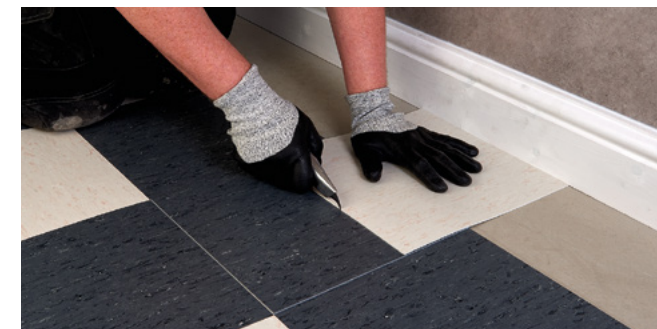
Figure 5 Measuring using an overlapping tile
