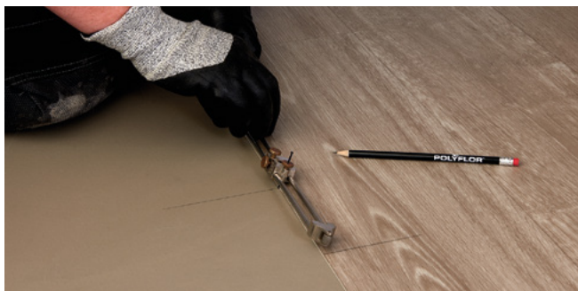
Figure 4 Scribing the wall profile
