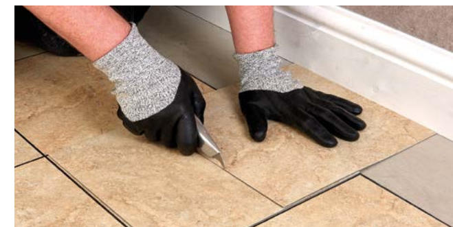
Figure 6 Measuring using an overlapping tile
