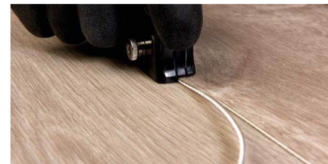
Figure 5 Cutting in the seams
