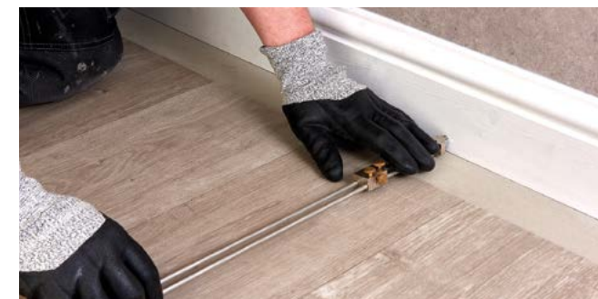
Figure 2 Scribing the wall profile
