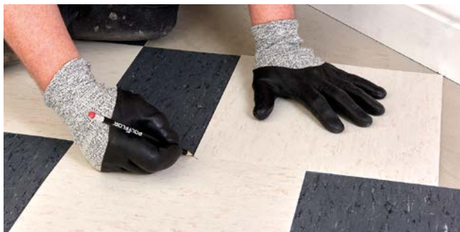
Figure 7 Marking the perimeter tiles (diagonal cut)
