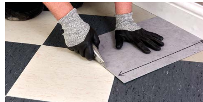
Figure 8 Cutting the perimeter tiles (diagonal cut)
