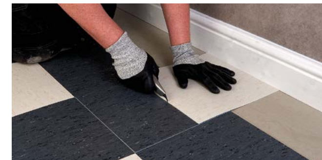
Figure 5 Measuring using an overlapping tile
