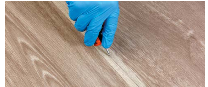
Figure 7 Cold welding
