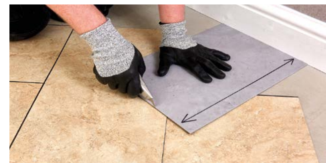
Figure 9 Cutting the perimeter tiles (diagonal cut)
