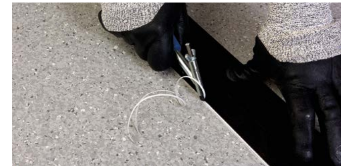
Figure 1 Grooving the seam
