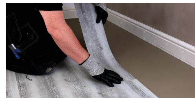
Figure 1 Setting planks out
