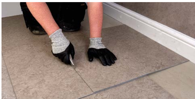
Figure 8 Measuring using an overlapping tile
