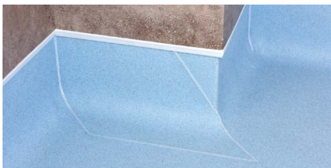
Figure 11 External corners 'wrap around method'
