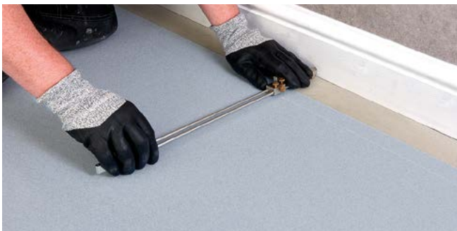
Figure 11 Scribing the wall profile
