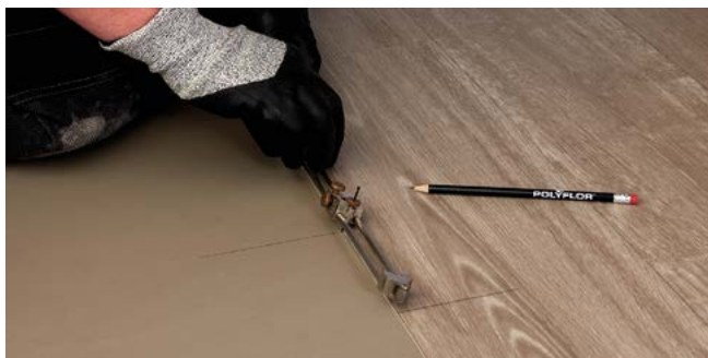
Figure 4 Scribing the wall profile
