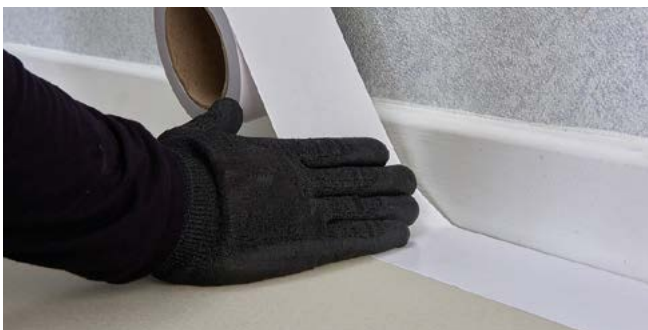
Figure 12 Use double sided Polyflor recommended tape
