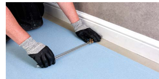
Figure 2 Scribing the wall profile
